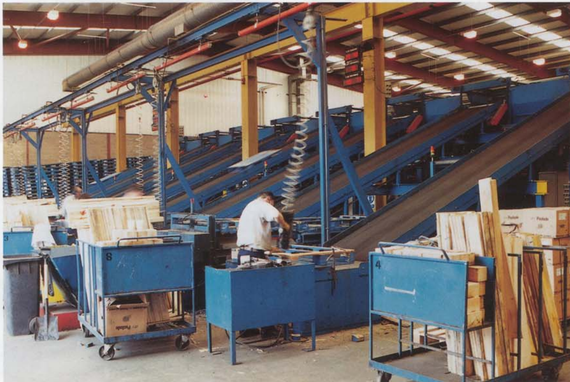
2 MULTIPLE INCLINED BELT CONVEYORS
