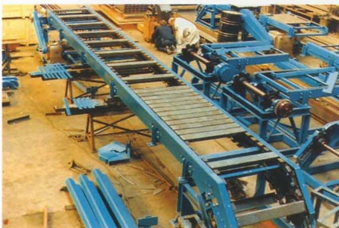
5. CONVEYORS UNDER ASSEMBLY
